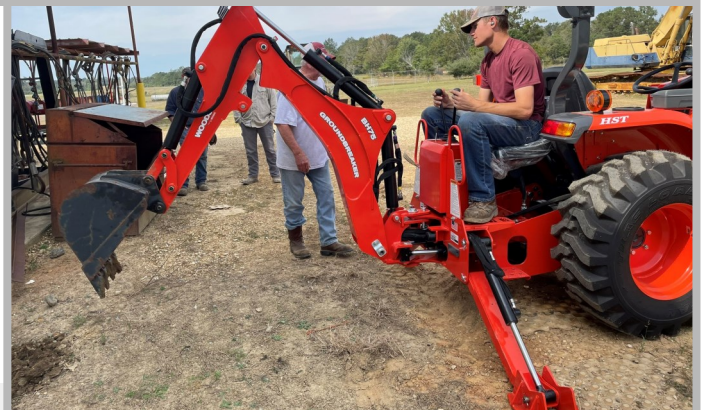
Logan Hanna repairing a water line
