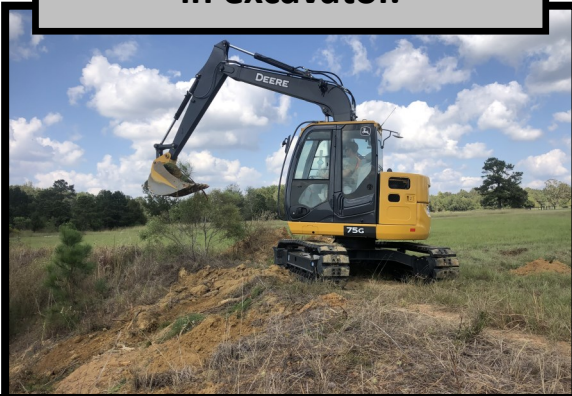
Apprentice Logan Hanna in excavator.
