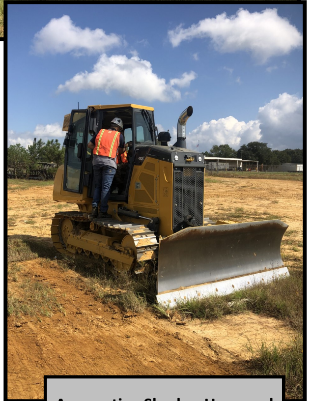
Apprentice Shaden Hammad helping Felicia Tanner on operating dozer.
