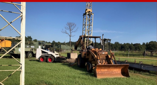
APPRENTICES JACK LEAGANS ON SKID STEER & COLLIN JOHNSON ON BACKHOE
