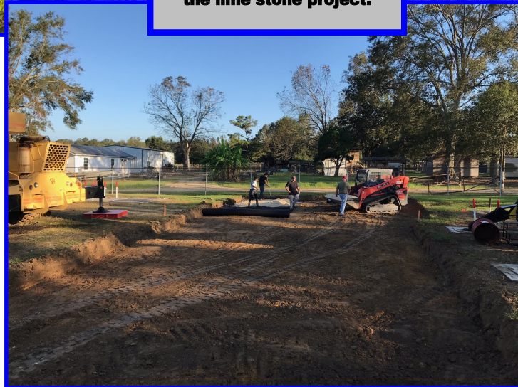
Instructor Leon Lemoine and apprentices working on the lime stone project.
