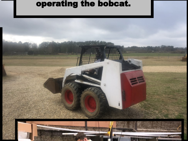
Apprentice Fredrick Roth operating the bobcat.
